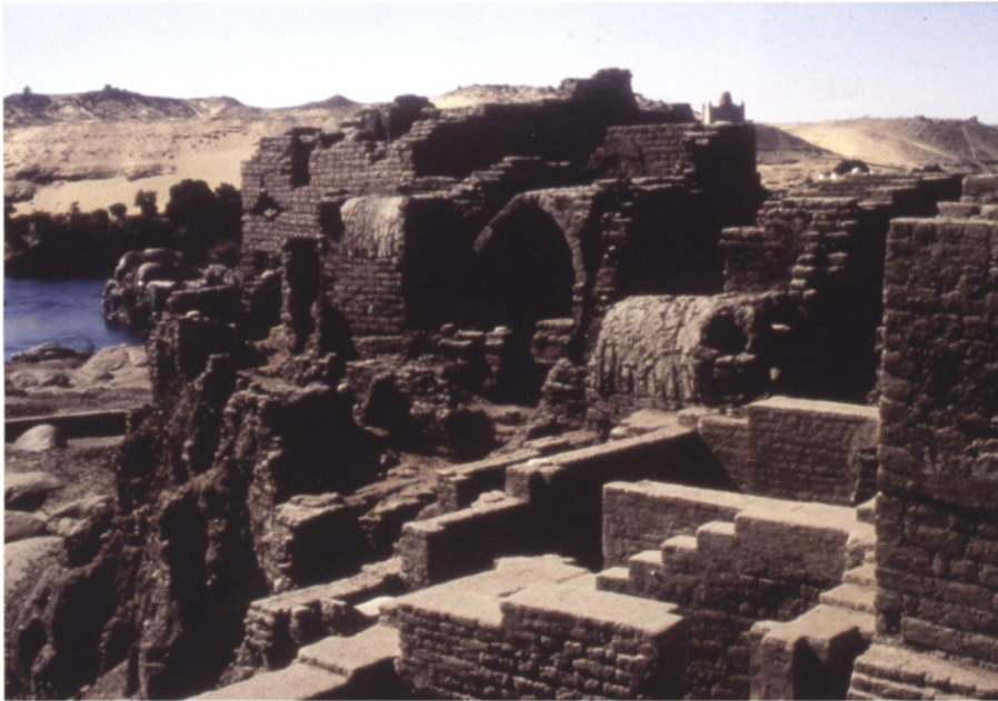
The multi-storied mudbrick Houses of the "Aramaean Quarter" at Elephantine discovered by the German Team date from the early part of the Persian period (525 to 404 BCE) and were structures with primitive finishes and beaten earth floors.
